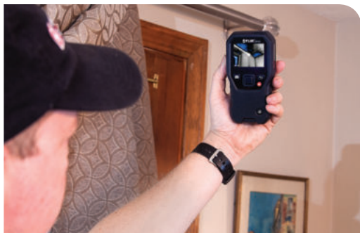
Scanning ceiling & wall joint for moisture issues
